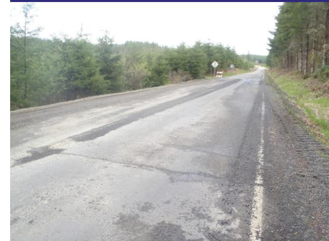
The Tower Road Slide Repair project will repair an existing slide at milepost 11.38. The slide will be repaired utilizing shear piles and replacing a damaged culvert.
