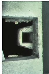
for easier maintenance. With the lids removed, inspect the inlet, outlet and crossover baffles to ensure they are present and not severely corroded. If the baffles are concrete and molded into the inside of the tank, the baffles should have venting holes that are unobstructed.
