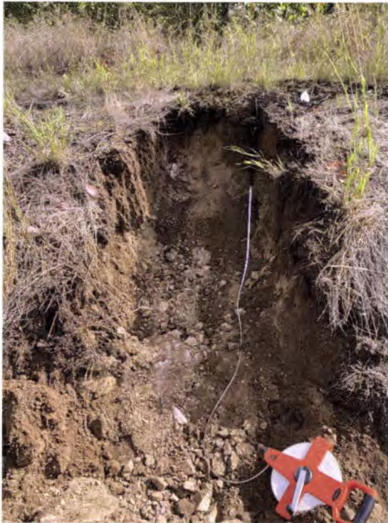
Photo 5: Test Pit TP-5
