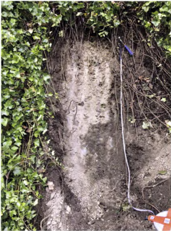
Photo 1: Test Pit TP-1
