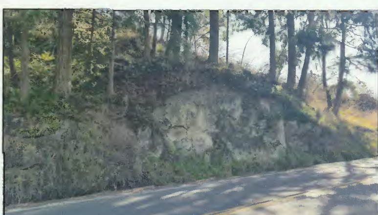
TAKEN ON WEST SIDE OF THE ROAD, LOOKING SOUTHEASTERLY AT THE ROCK CLIFF (PHOTO TAKEN 3/12/2020)
