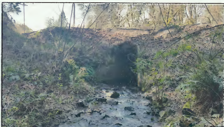
TAKEN ON EAST SIDE OF THE ROAD, UPSTREAM FROM THE CULVERT, LOOKING WEST AT THE BOX INLET (PHOTO TAKEN 3/12/2020)
