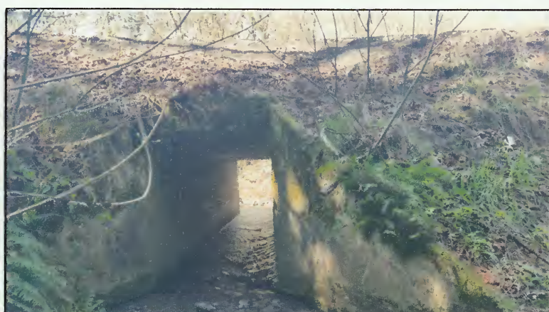
TAKEN AT THE INLET OF THE CULVERT, LOOKING WEST THROUGH THE BOX (PHOTO TAKEN 3/12/2020)
