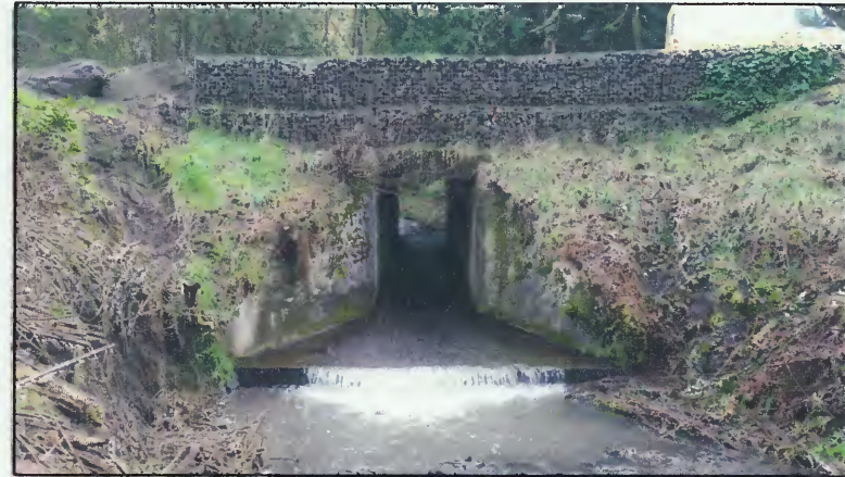
TAKEN WEST OF THE BOX CULVERT, LOOKING EAST AT THE GABION WALL AND OUTLET OF THE CULVERT. (PHOTO TAKEN IN 2015 WITH BRUSH CLEARED. BRUSH HAS GROWN BACK IN 2021 BUT THE GROUND CONDITIONS APPEAR UNCHANGED)
