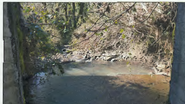
TAKEN FROM INSIDE THE BOX CULVERT AT THE WEST END, LOOKING WEST AT THE OUTFALL. (TAKEN IN 2020)
