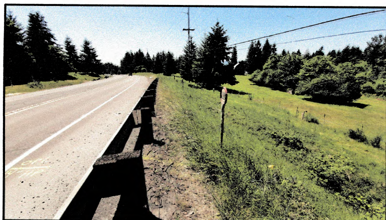
TAKEN FROM NEAR THE CENTER OF THE GUARD RAIL ON THE NORTH SIDE OF SR504, LOOKING SOUTHWESTERLY ALONG SR504.
