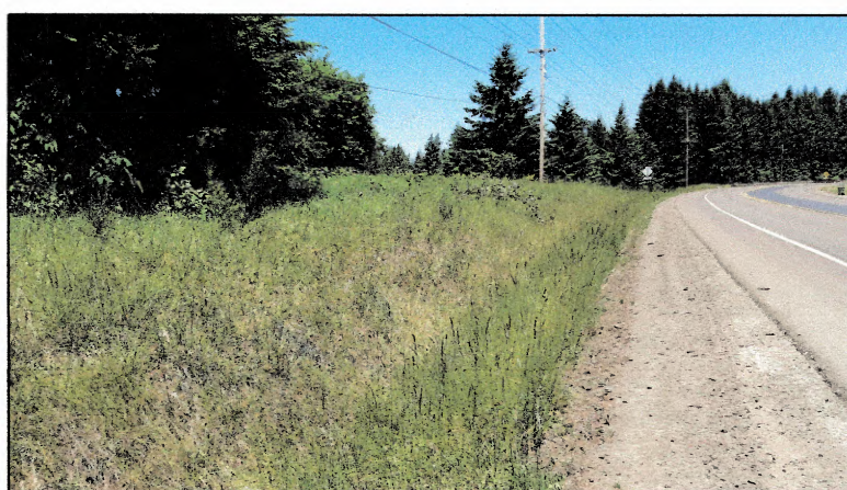
TAKEN ON THE WEST SIDE OF SR504, JUST NORTH OF KROLL ROAD, LOOKING NORTHERLY AT THE EDGE OF ROADWAY AND CUT BANK
