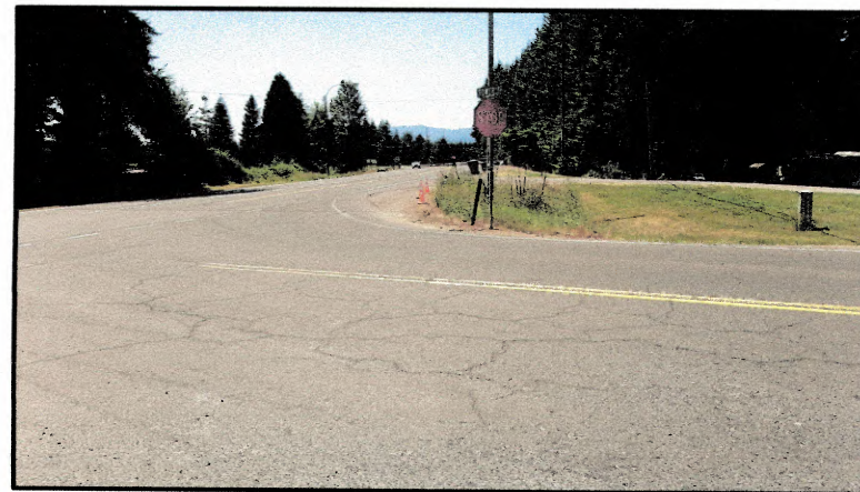
TAKEN FROM EASTERLY EDGE OF TOWER ROAD, NEAR ITS INTERSECTION WITH SR504, LOOKING WESTERLY DOWN SR504.
