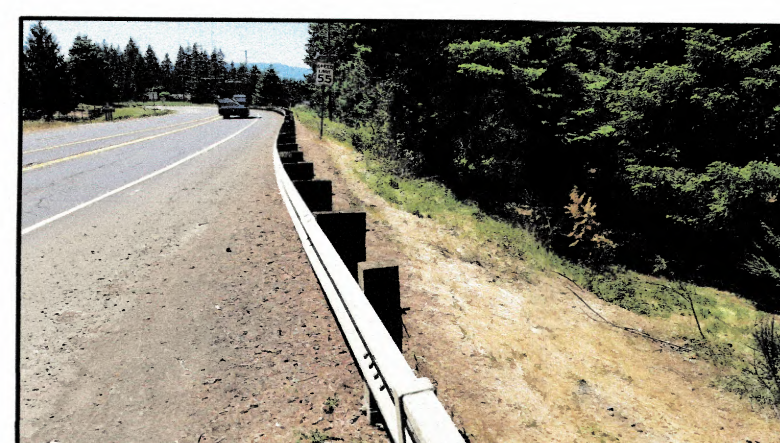
TAKEN NEAR EASTERLY END OF GUARDRAIL ON NORTHERLY SIDE OF SR504, LOOKING WESTERLY ALONG SR504.
