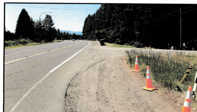
TAKEN FROM NORTHERLY EDGE OF SR504, NEAR CONTROL POINT #12, LOOKING WESTERLY ALONG SR504.
