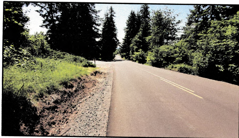
TAKEN FROM THE SOUTHEASTERLY EDGE OF SCHAFFRAN ROAD, JUST NORTHEASTERLY OF THE KOA ENTRANCE ROAD, LOOKING SOUTHWESTERLY DOWN SCHAFFRAN.
