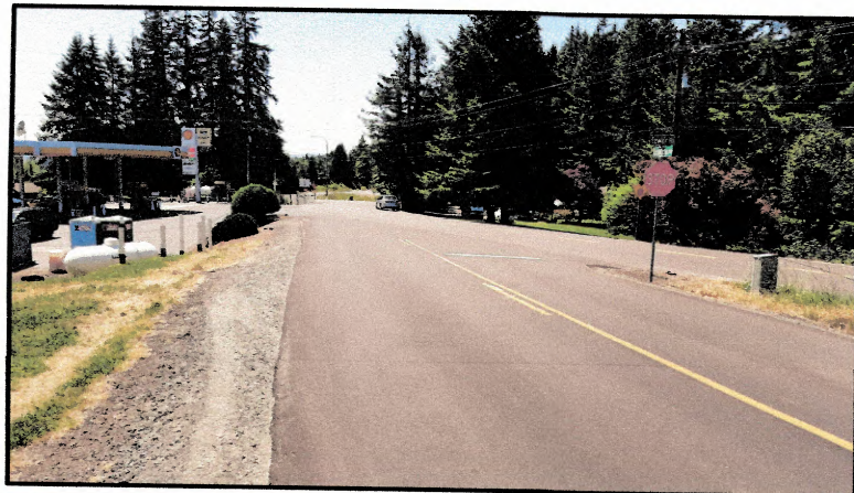
TAKEN FROM SOUTHEASTERLY SIDE OF SCHAFFRAN ROAD, LOOKING SOUTHWESTERLY TOWARDS INTERSECTION WITH TOWER ROAD.
