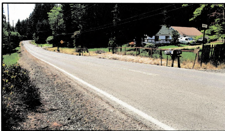
TAKEN EAST OF JUANITA WAY, LOOKING SOUTHWESTERLY AT THE ROADWAY AND FENCES
