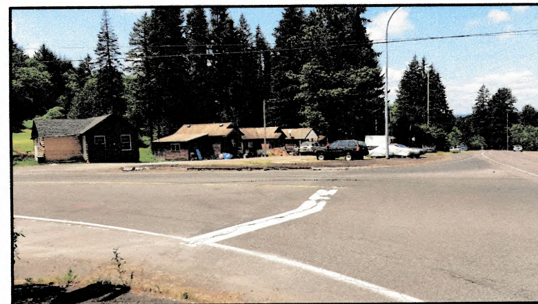
TAKEN AT SOUTHEAST CORNER OF INTERSECTION, LOOKING WESTERLY AT THE ROAD AND CABINS
