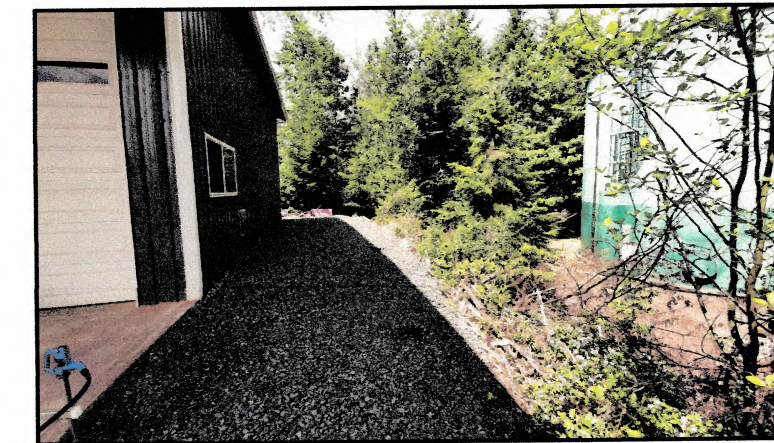
TAKEN SOUTHEAST OF THE WATER TOWER, LOOKING WEST AT THE NEIGHBORING SHOP AND ENCROACHING GRAVEL
