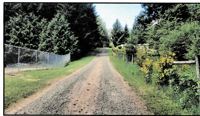
TAKEN AT THE CENTERLINE OF THE GRAVEL DRIVEWAY, LOOKING WEST AT THE FENCES AND DRIVEWAY
