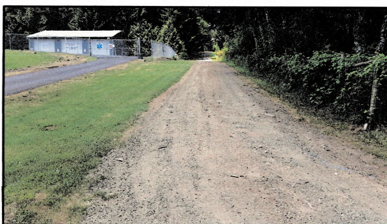
TAKEN AT THE ENTRANCE OF THE GRAVEL DRIVEWAY TO THE WATER TANK, LOOKING WEST AT THE DRIVEWAY
