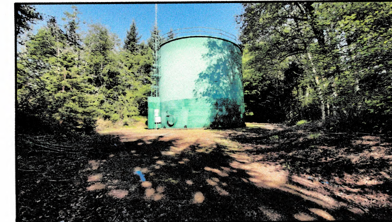
TAKEN AT THE GATE NEAR THE WEST END OF THE DRIVEWAY, LOOKING WEST AT THE WATER TOWER
