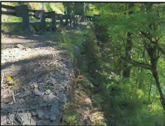
TAKEN ON THE SOUTHWESTERLY SIDE OF THE ROAD, LOOKING SOUTHEASTERLY ALONG THE GABION WALL
