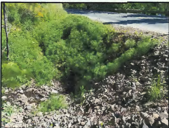
TAKEN ON NORTHEASTERLY SIDE OF THE ROAD, LOOKING SOUTHERLY AT THE CULVERT INLET (BEFORE BEING BURIED IN 2017)
