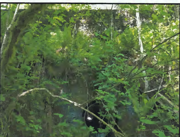
TAKEN ON THE SOUTHWESTERLY SIDE OF THE ROAD, LOOKING NORTHEASTERLY AT THE CULVERT OUTLET
