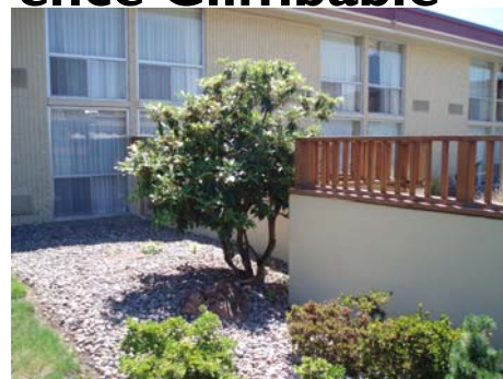
Bushes near fences such as this one should be evaluated to determine if they are climbable
